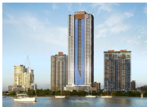
Boral is supplying concrete for Meriton's Sundale Apartments: a 55-storey residential tower in Southport, Gold Coast, Queensland
